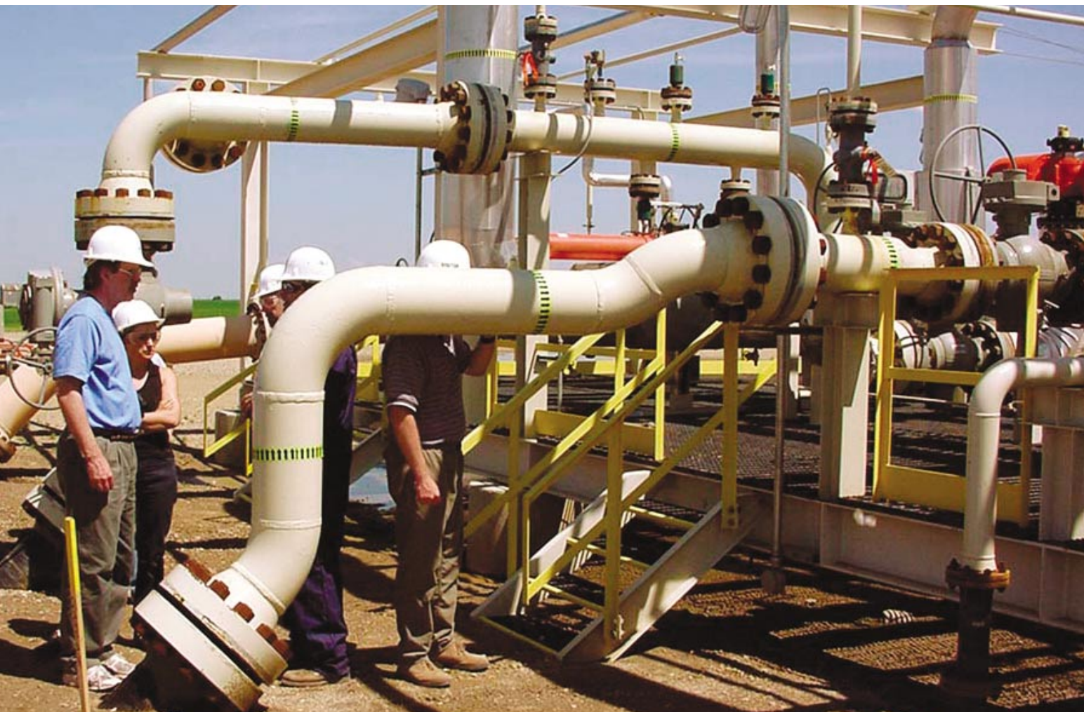
Above: Weyburn CO 2 Monitoring and Storage Project researchers and sponsors tour the facility where the main CO 2 pipeline comes into the Weyburn field from Beulah, North Dakota.
